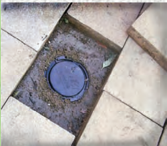
Installation under pavers
