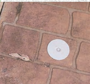
Installation through concrete.
